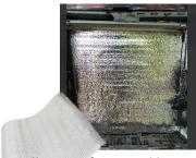
Installation of internal lining for thermal insulation and reflection of grow lights
